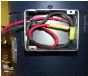
With the Leeson Motors (Dark blue in color), the direction can be changed by cutting the leads inside the junction box located on the side of the motor. Re-connection the red wire to the black wire and the black wire to the red wire. As shown in the lower picture Motors with the fuse holder you will need to remove the cover completely in order to get to the red and black wires. Be sure to use the enclosed 10 gauge connectors.
