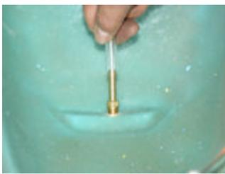
Install the 17" piece of clear vinyl hose on the barb fitting. Install the hose clamp to hold the hose in place.
